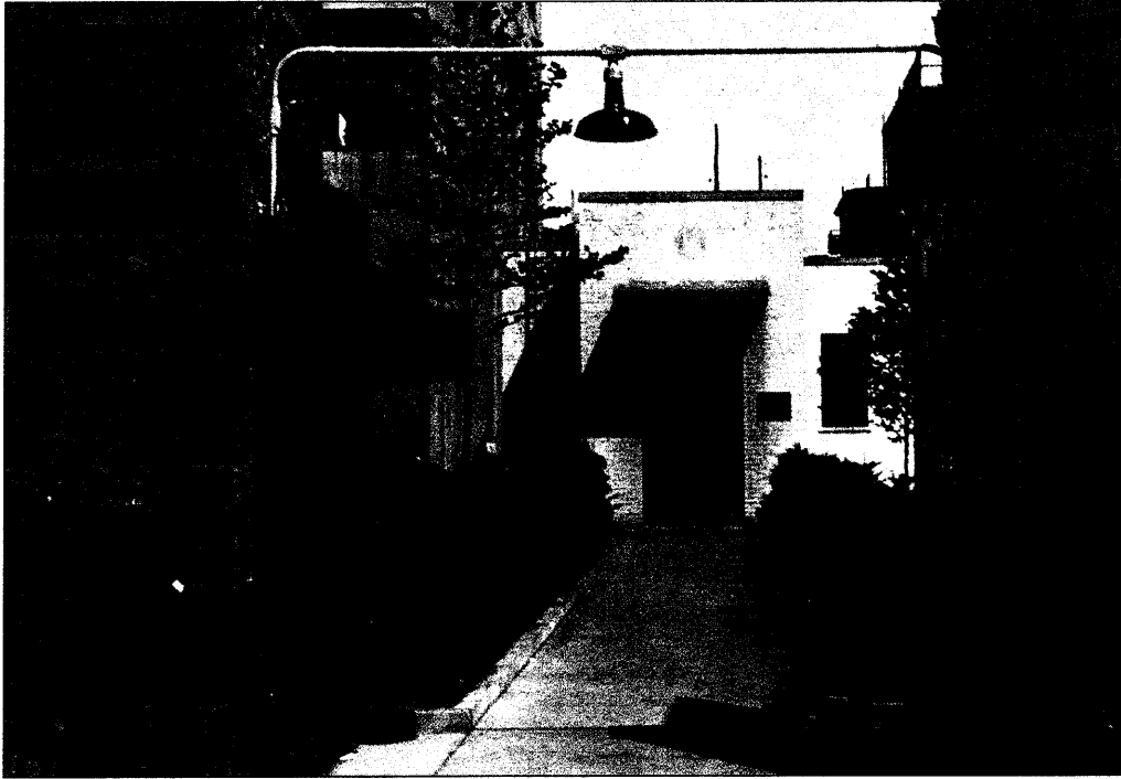
In 1933, Cornelia E. and Jennie A. Donnellon donated their residence at 116 Pacific Street as a recreation center for students. The basement of the building was converted into a cafeteria for students and faculty. The cafeteria was later enlarged and given the name the Open Gate.
